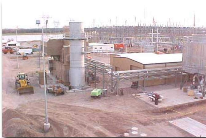
Recent Construction at Horseshoe Lake Facility
