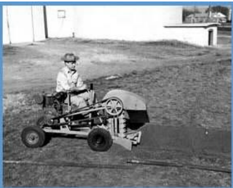
Ed Malzahn (ca. 1950) digs a 4 x 24 inch trench using the DWP trencher for the installation of a water line. ASME will designate the first trencher as an ASME landmark on Dec. 16, at Charles Machine Works, Perry, Oklahoma.
