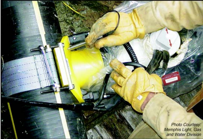
Above: A construction worker installs a Kerotest POLYBALL™ valve into a new piping system.
